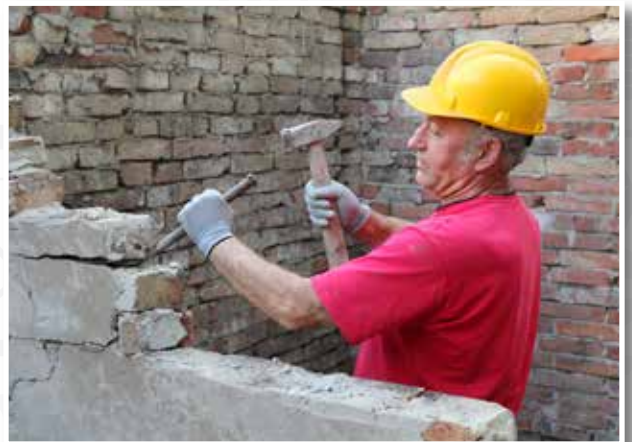
Chipping mortar without a mask or safety goggles
