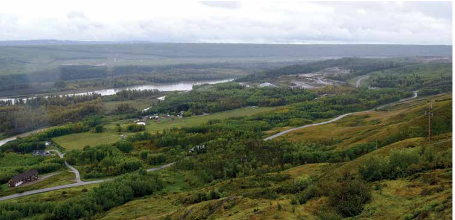
Site C Dam construction site | Photo by Jeffrey Wynne
